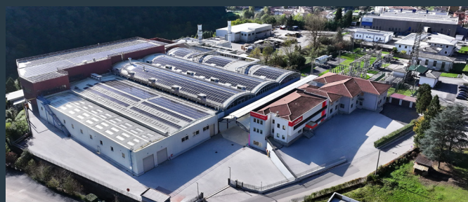
PLANT V1 VESTONE (BS) Production site for extruded and designer radiators.
